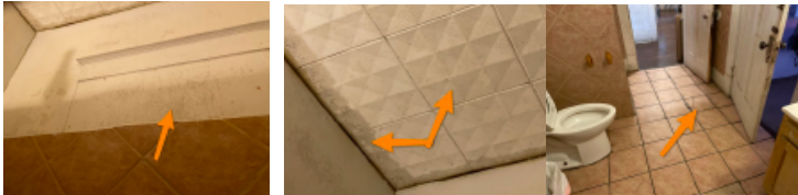
Fungal growth in bathroom, due to improper ventilation
